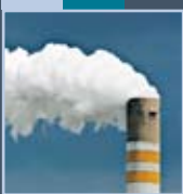
AIR POLLUTION CONTROL
